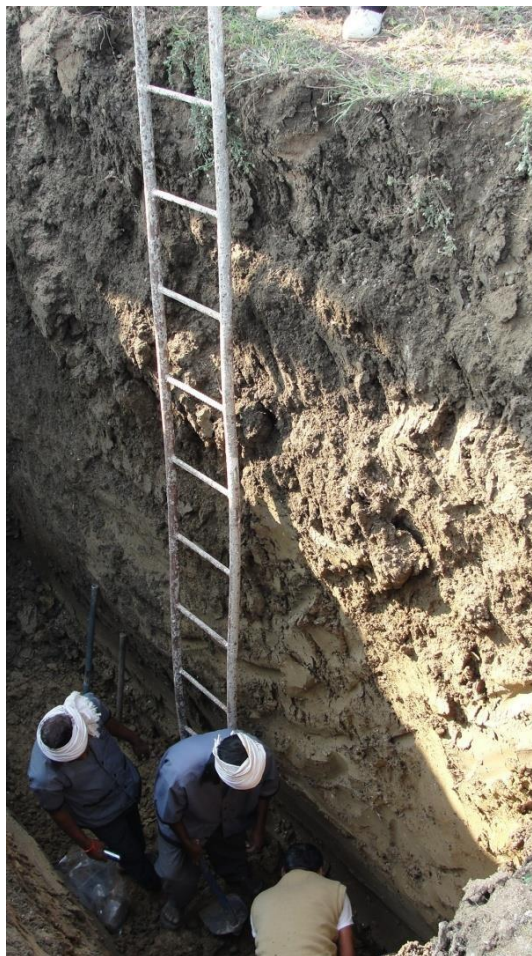
Fig. 12 Geotechnical Investigations in IIIT, Basar
