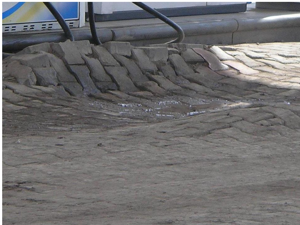
Fig. 16 Forensic GT Investigation of Distress of floor of a Petroleum Retail Outlet
