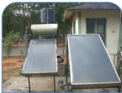
Solar Water Heater-Flat Plate Collector
