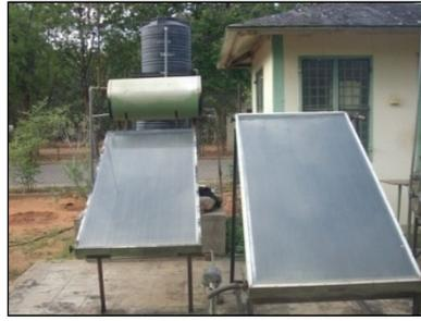
Solar Water Heater-Flat Plate Collector
